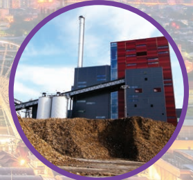
Community Power Plant
