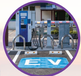
EV Charging Station
